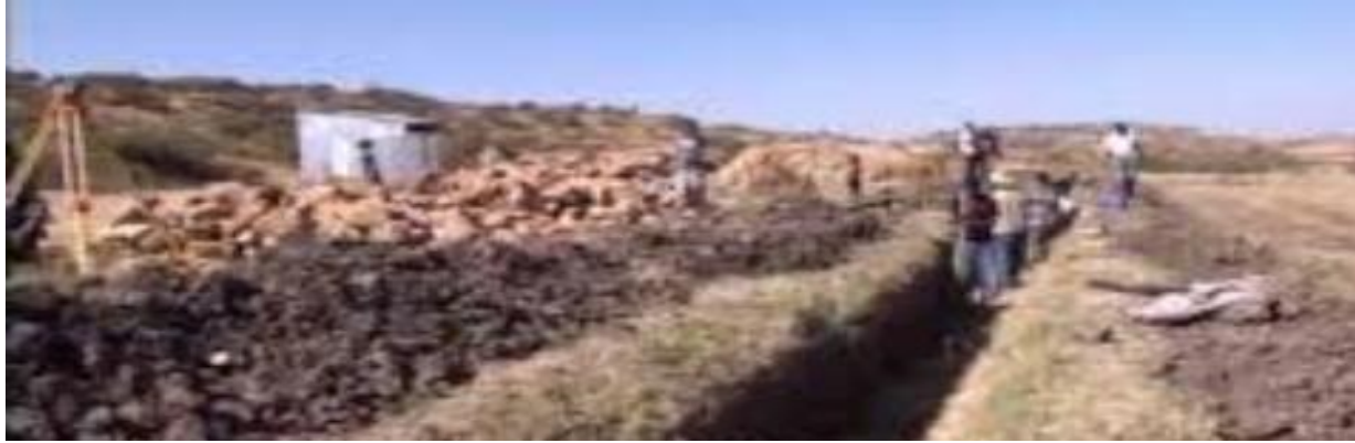
Figure 3 Construction of canal structures in spate scheme
