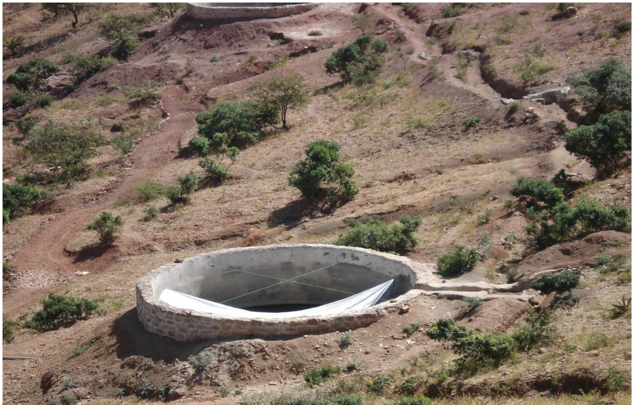
Figure 10 Series of underground tankers at Kola Tembian Wereda
