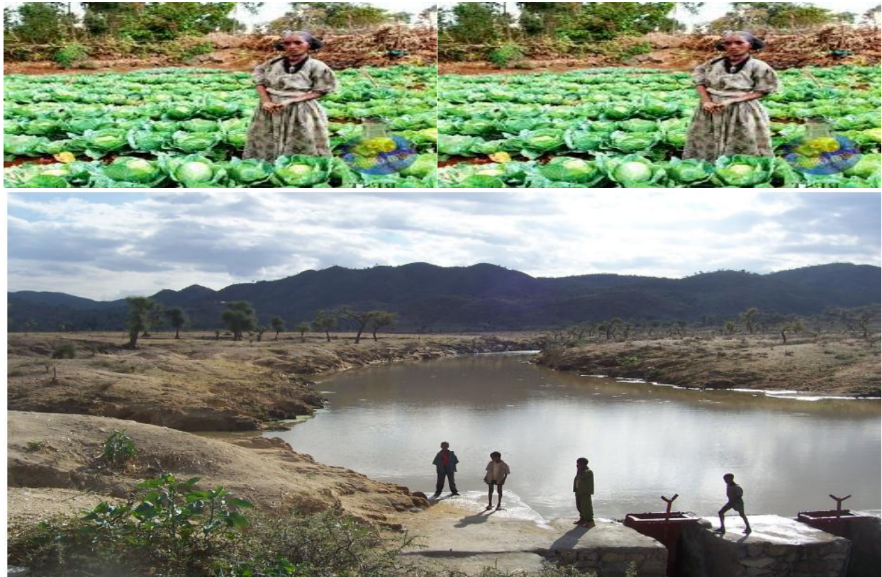
Figure 12 Check dams at Merebe Leke
