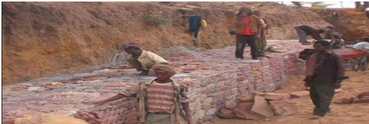
Figure 2Construction of check dams in Ahferomwereda in the area of food insecure
